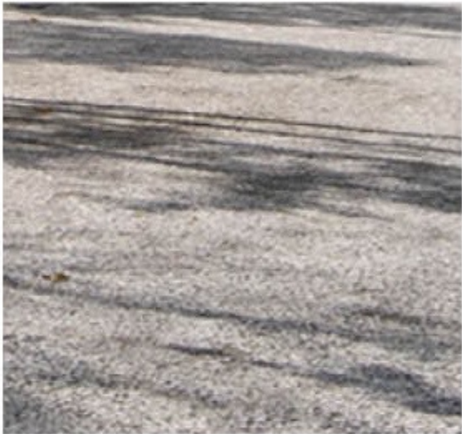
Ground Surface | Stabilized Granite
