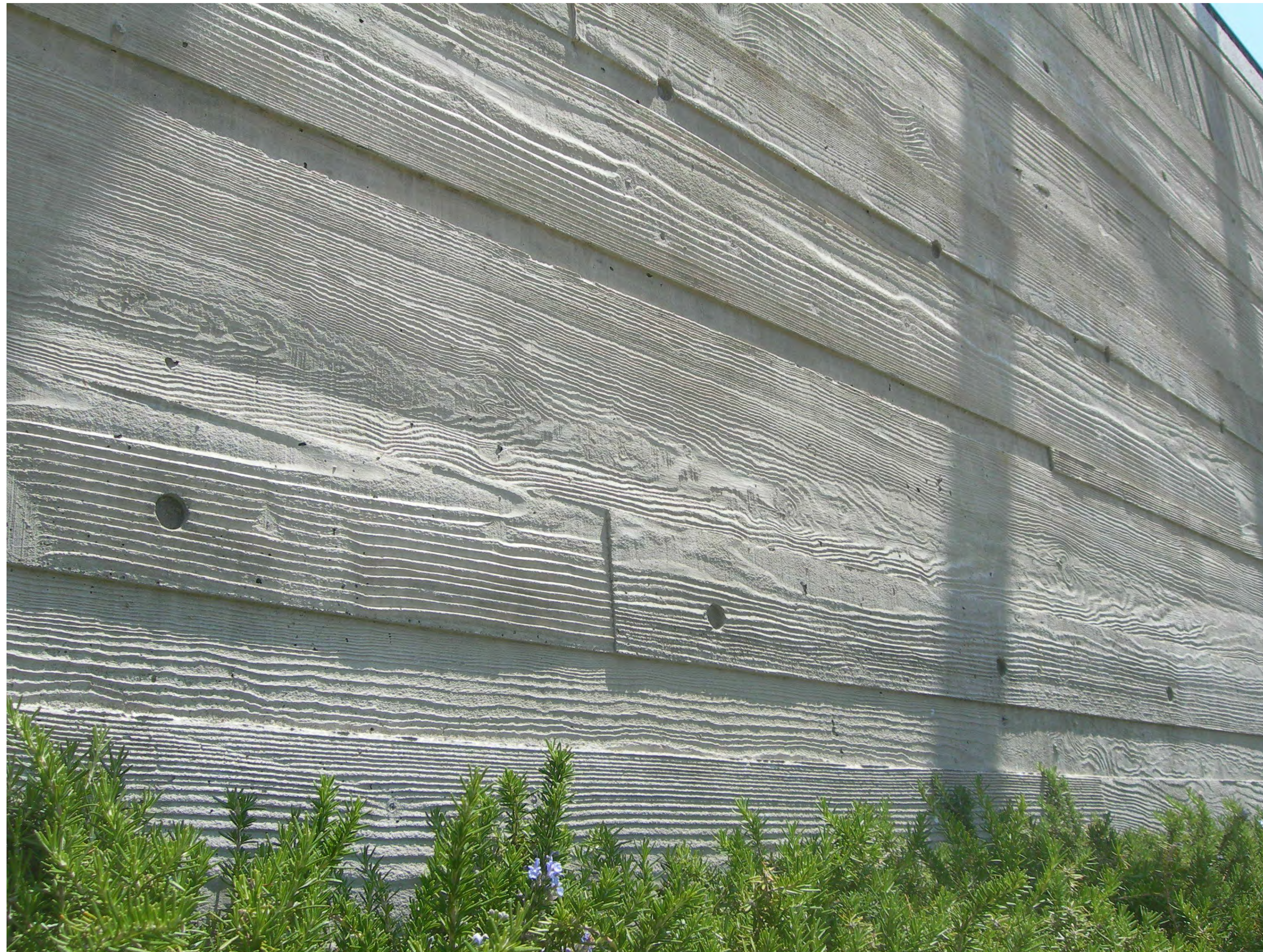
Board Formed Concrete
