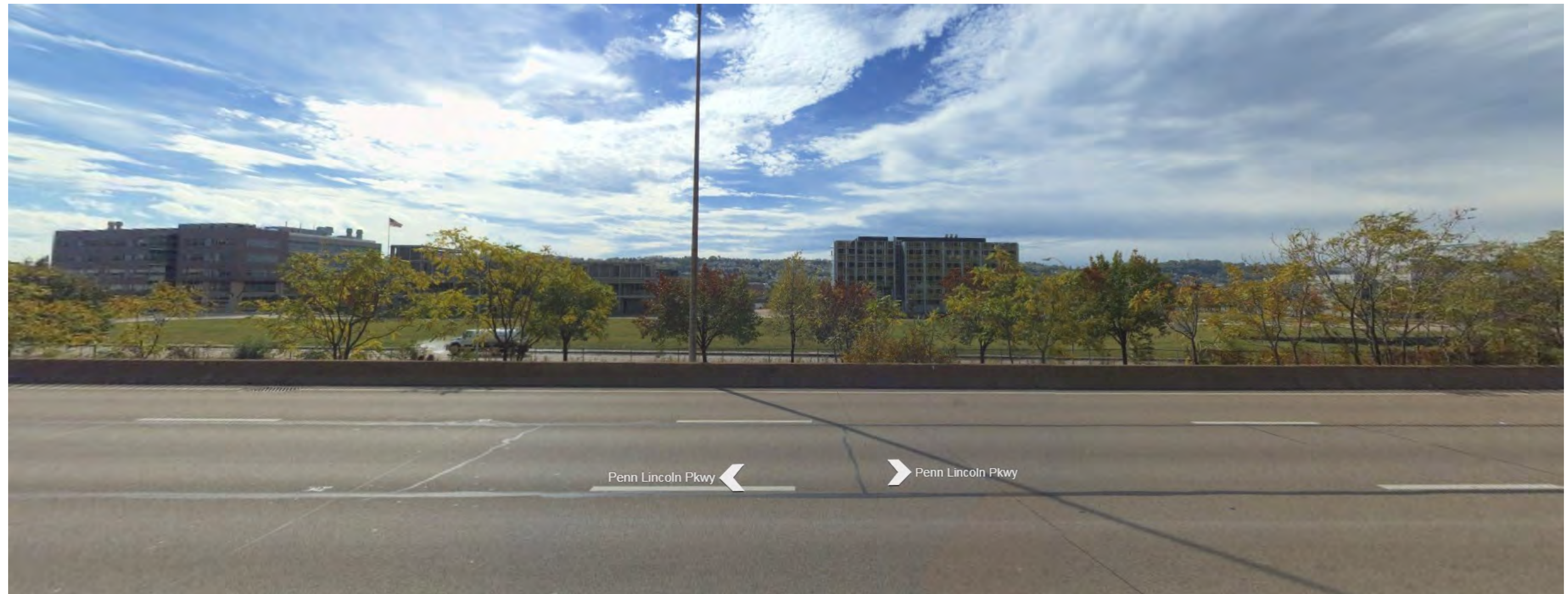
View Of Site + Adjacent Buildings From Parkway
