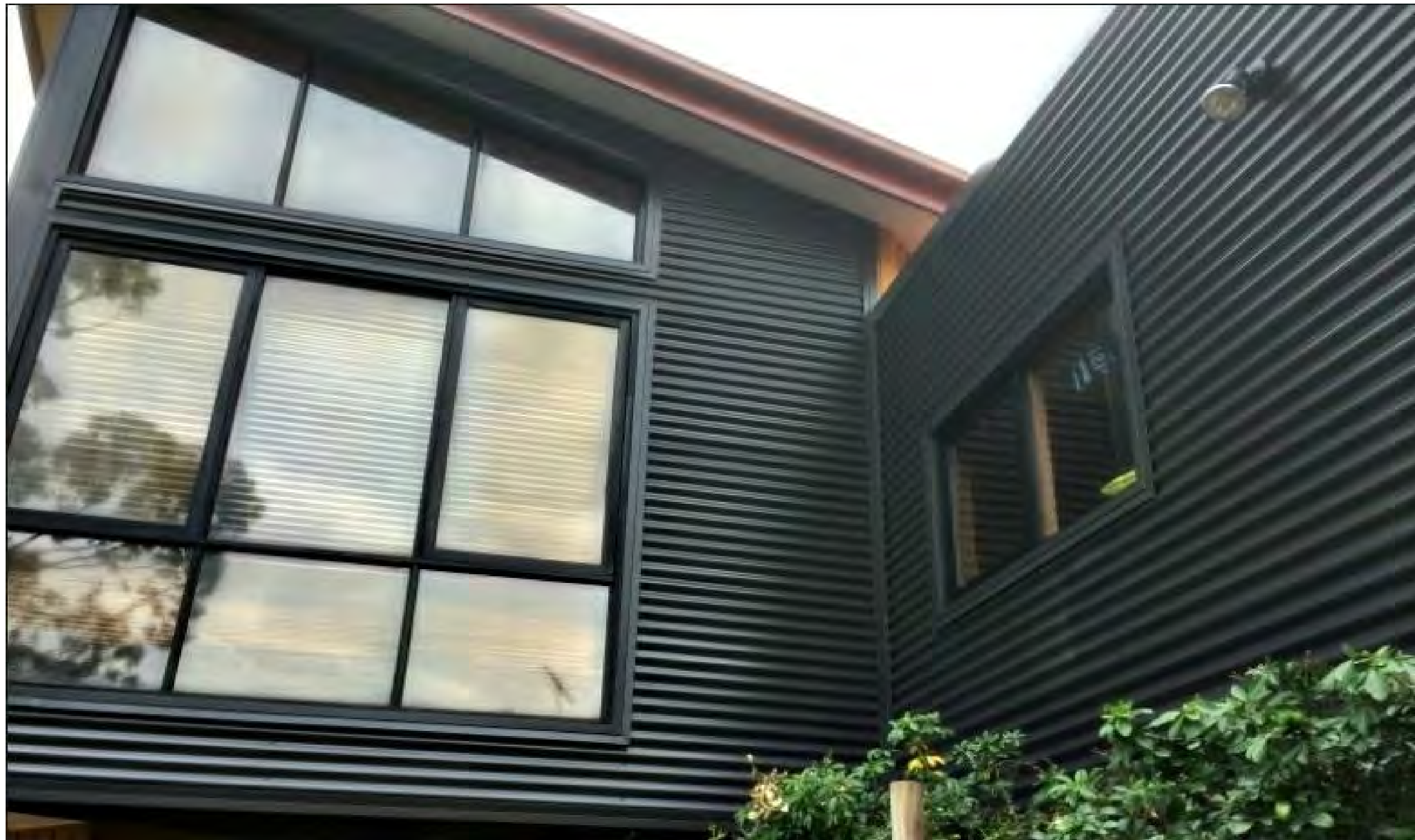
Heavy Corrugated Metal panels
