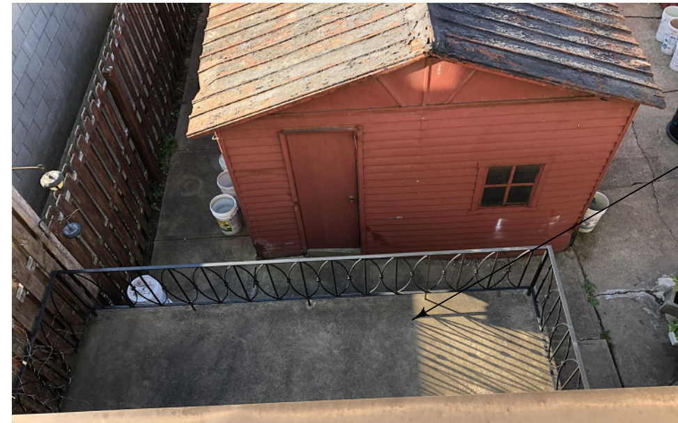
PORCH TO BE REDUCED TO ORIGINAL DEPTH (FLUSH WITH BACK OF HOUSE)
