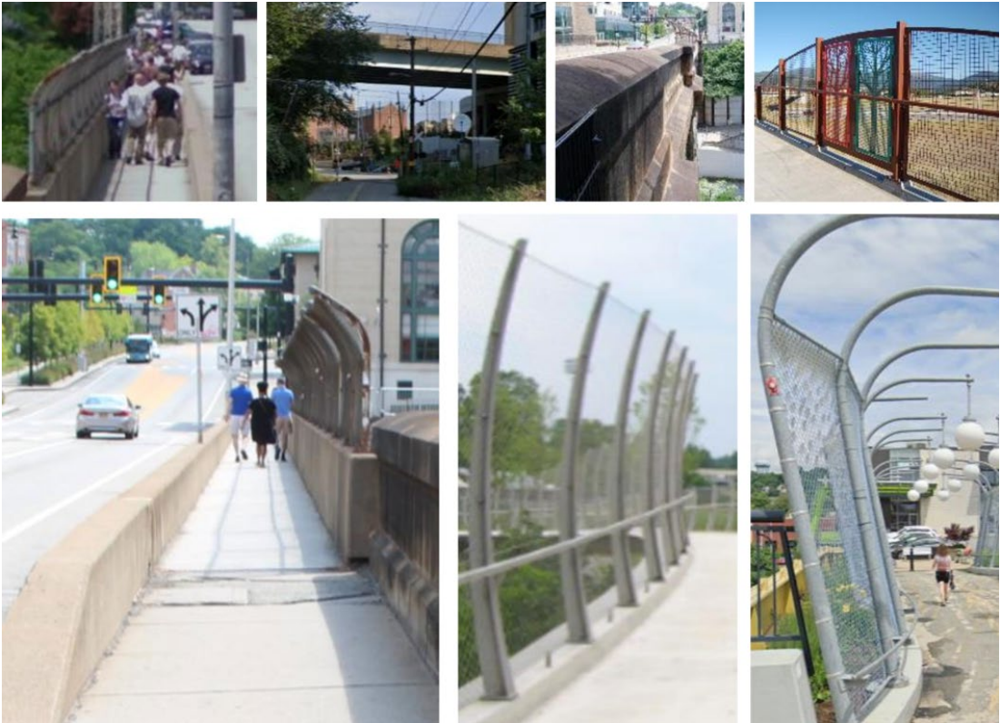
Improve Aesthetics of Fencing and Widen Sidewalk on Forbes Bridge
